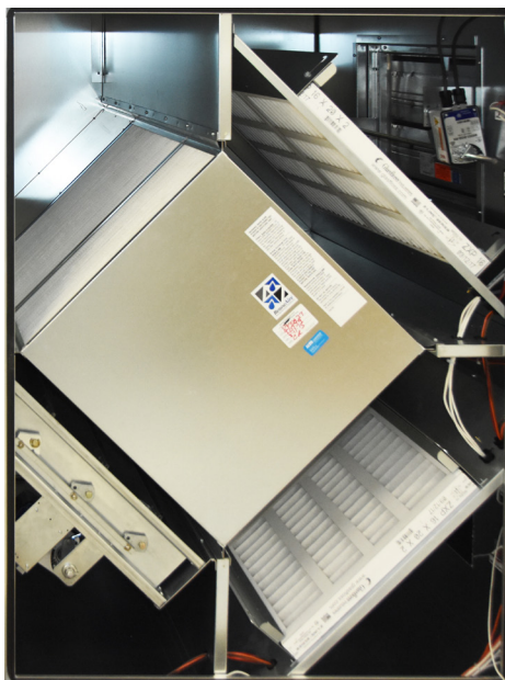
FIGURE 7.1.0 END VIEW OF CORE SUPPORT ASSEMBLY
