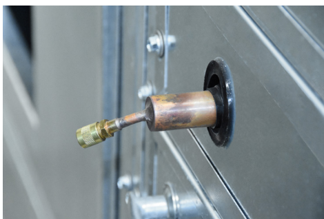
FIGURE 5.5.0 SUCTION LINE FOR DX COIL
