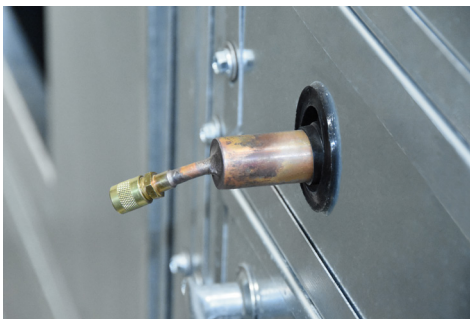
FIGURE 5.7.0 SUCTION LINE FOR DX COIL
