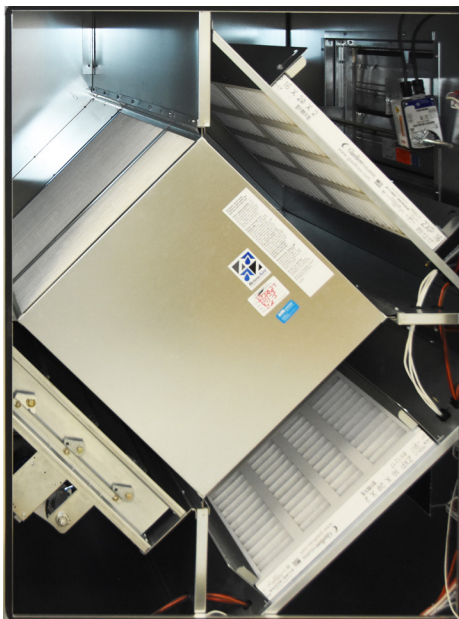
FIGURE 7.1.0 END VIEW OF CORE SUPPORT ASSEMBLY
